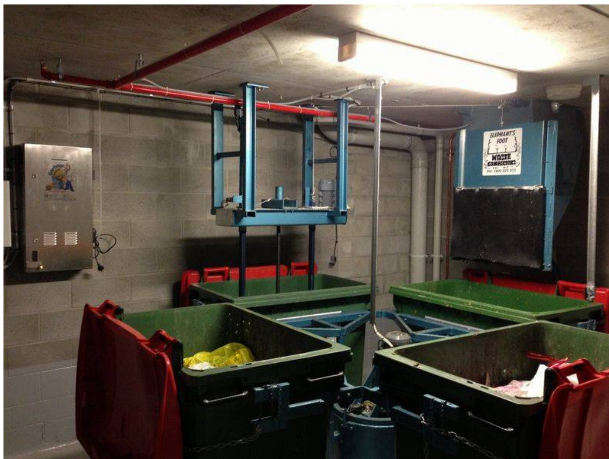
Figure 8 A three (3) bin waste carousel with compactor will be used.
